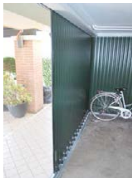
Vista interna Internal view
